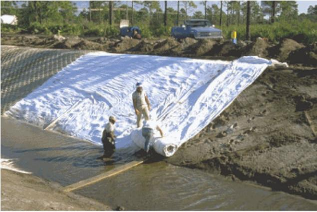
Once positioned, the upper edge of the panel is folded into the anchor trench atop the slope. The extra fabric provided for contraction during pumping should be accumulated and held at the top of the slope and gradually released as the panel is filled. Adjacent panels are joined by field sewing or zippering the double-layer fabric forms, bottom edge to bottom edge, and top edge to top edge.
